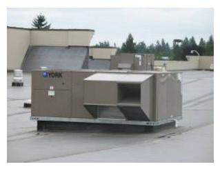
In order for the economizer to function, the HVAC system needs to be on and in the first stage of cooling. This is most easily accomplished by connecting a jumper wire at the terminal strip. **This should be done by the installer in accordance with the manufacturer's recommendations**. If the outdoor temperature is below 60°F, the unit's outside air damper should slowly modulate open. If it doesn't, try cooling the outside air sensor with some ice in a plastic bag or by spraying it with
