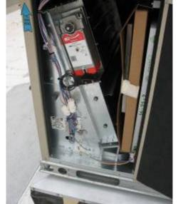
The economizer modulates exhaust air, return air and outside air dampers to maintain the mixed air temperature at its setpoint (around 60°F.) The action of the outside air damper and relief damper, if there is one, should always be opposite that of the return air damper. When the outside air is cool enough to cool the building (about 60°F or less) and there is a call for cooling, the
